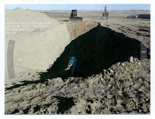
Report Photo #8 Subsoil from Security Trench Placed on Topsoil
